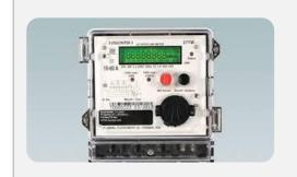
120 Nos. of Energy meters are provided in energy intensive machines for micro level monitoring
